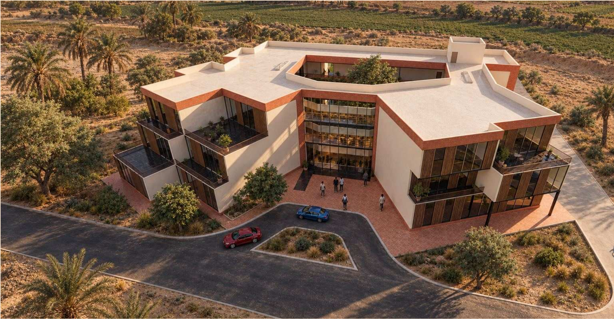
03.01 Aerial view of the courtyard
